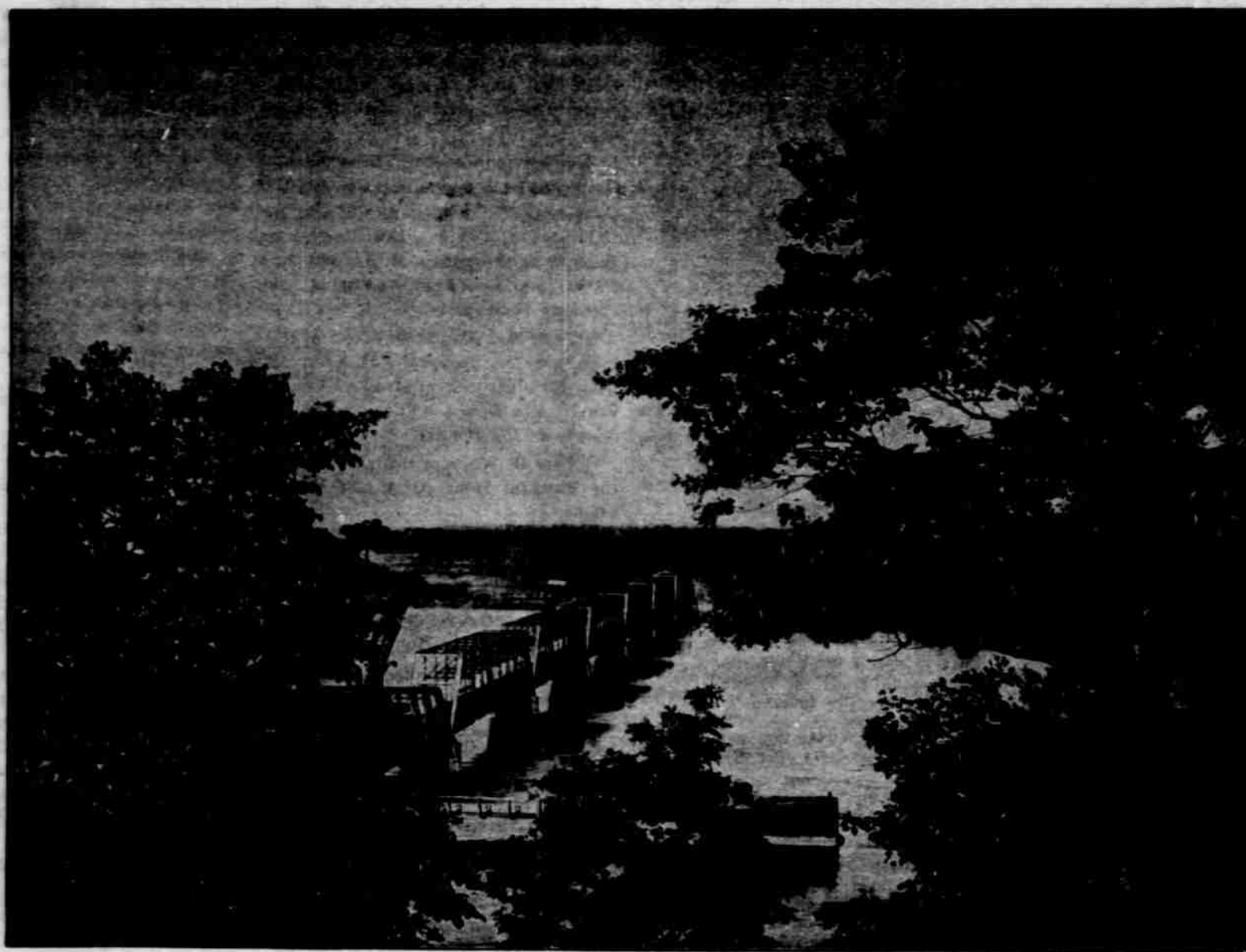
Bridge over the Mississippi River at Burlington, Iowa, on the G. B. & Q. Railroad.
