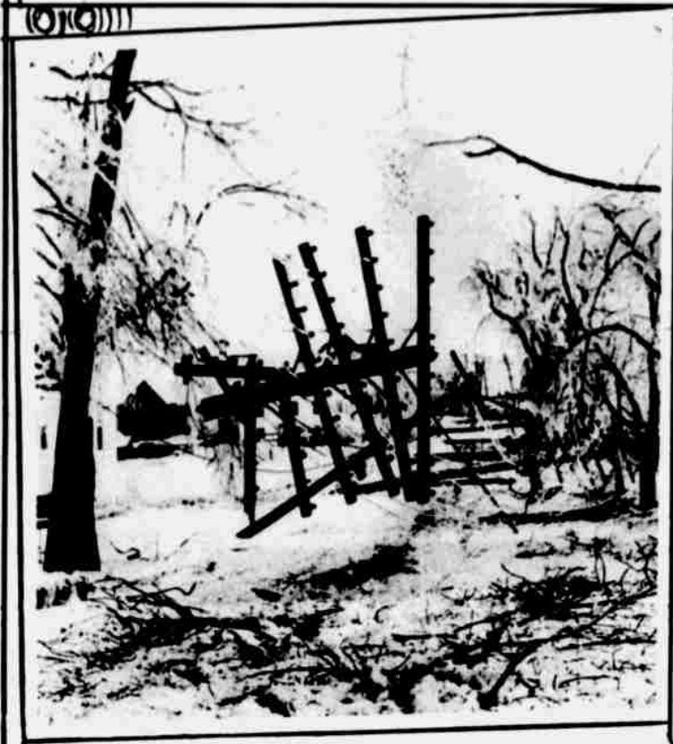
Fighting sleet is the hardest battle the Northwestern Bell Telephone company wages in Nebraska during the winter and early spring, company officials say. A glance at these pictures will demonstrate why phone service is not always up to standard after a hard sleet storm. The photographs were taken in the vicinity of Grand Island, Neb., just after the storm of March 18. Upper picture shows how wires were pulled down by weight of the ice. In the lower right picture a heavy pole has snapped under the strain and is standing on its head. Lower left shows an intricate tangle of crossed wires linemen had to contend with just outside Grand Island.
