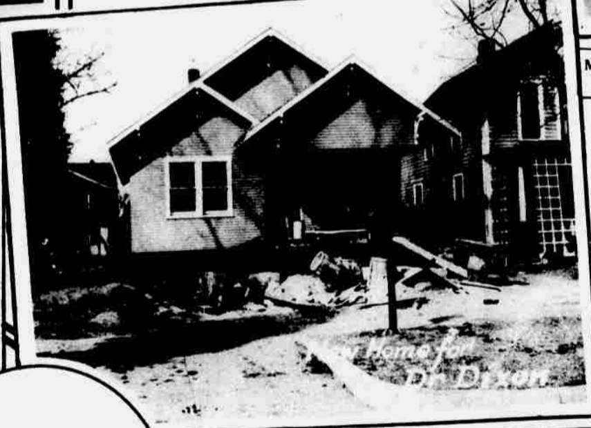
Typical of forty houses now under construction with aid of Home Builders' Fund.
