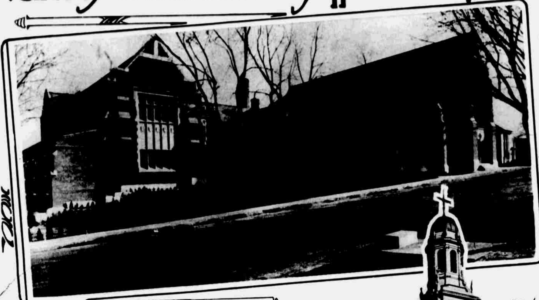
The First Central Congregational church, Thirty-sixth and Harney streets, is a fine example of Tudor Gothic.
