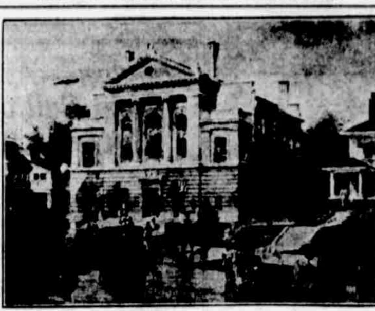
This is the new edifice of the Second Church of Christ, Scientist, Forty-first and Davenport streets, as it will look when completed next fall. The basement and Sunday school room were completed in 1916. Work on the superstructure will begin this spring.
