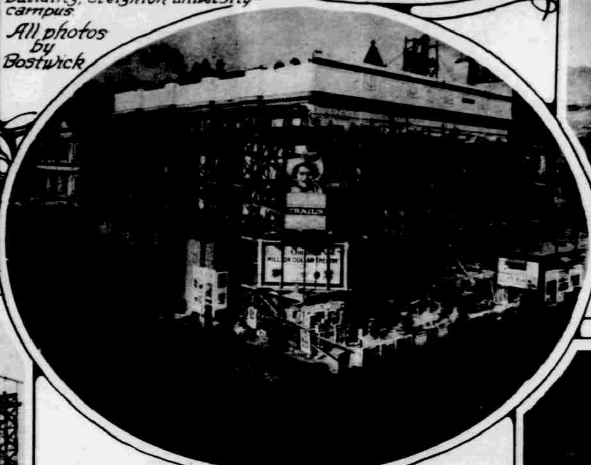
Workmen are putting the finishing touches on the World theater building, Fifteenth and Douglas sts
