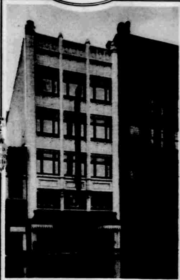
The new Hotzberg building, 1519-21 Douglas street.
