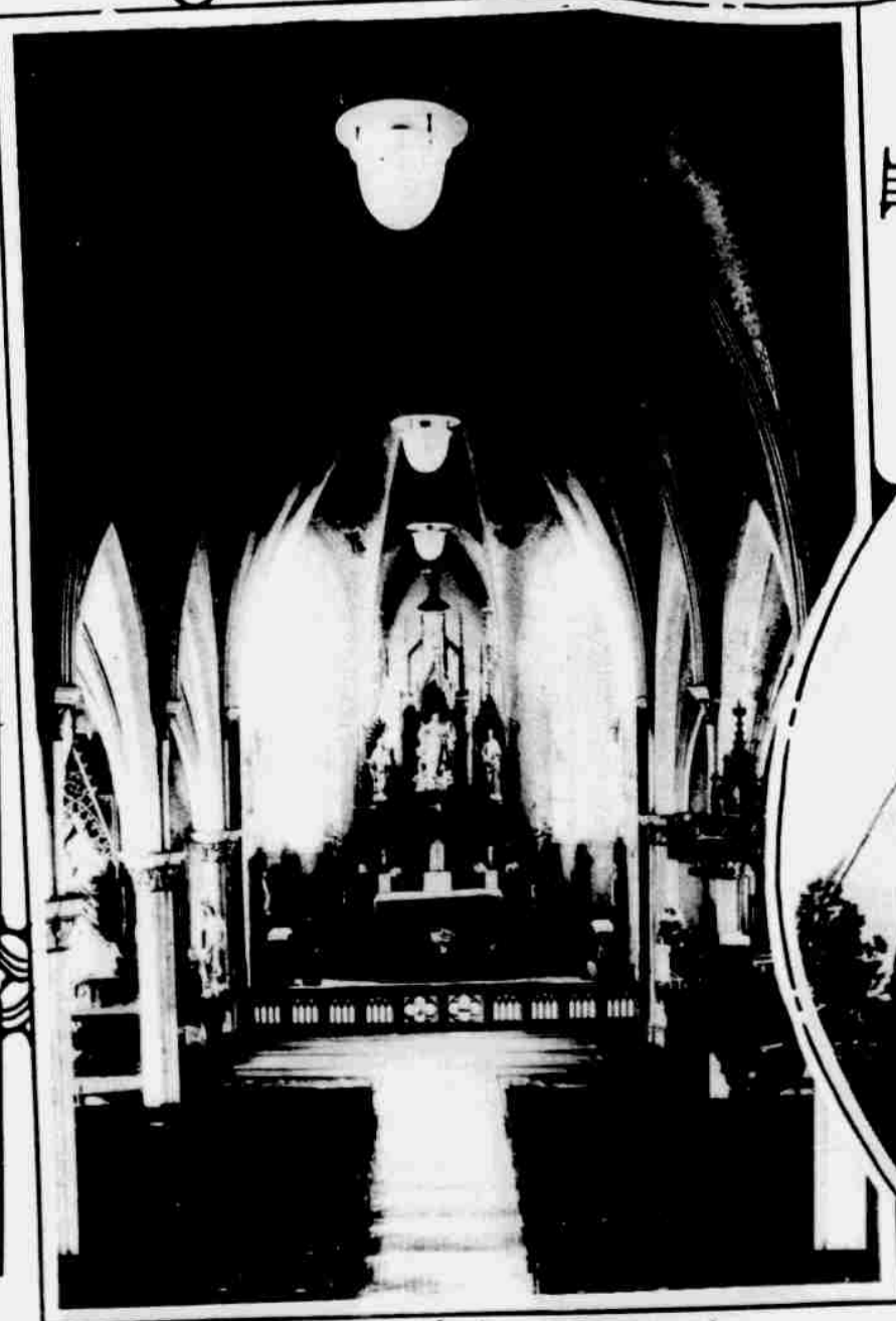
Interior St. Mary's Catholic Church, West Point
