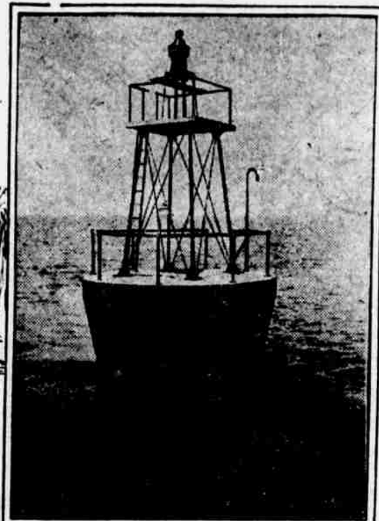
A light carrying steel caisson, Chesapeake Bay. A bell is to be mounted on it
