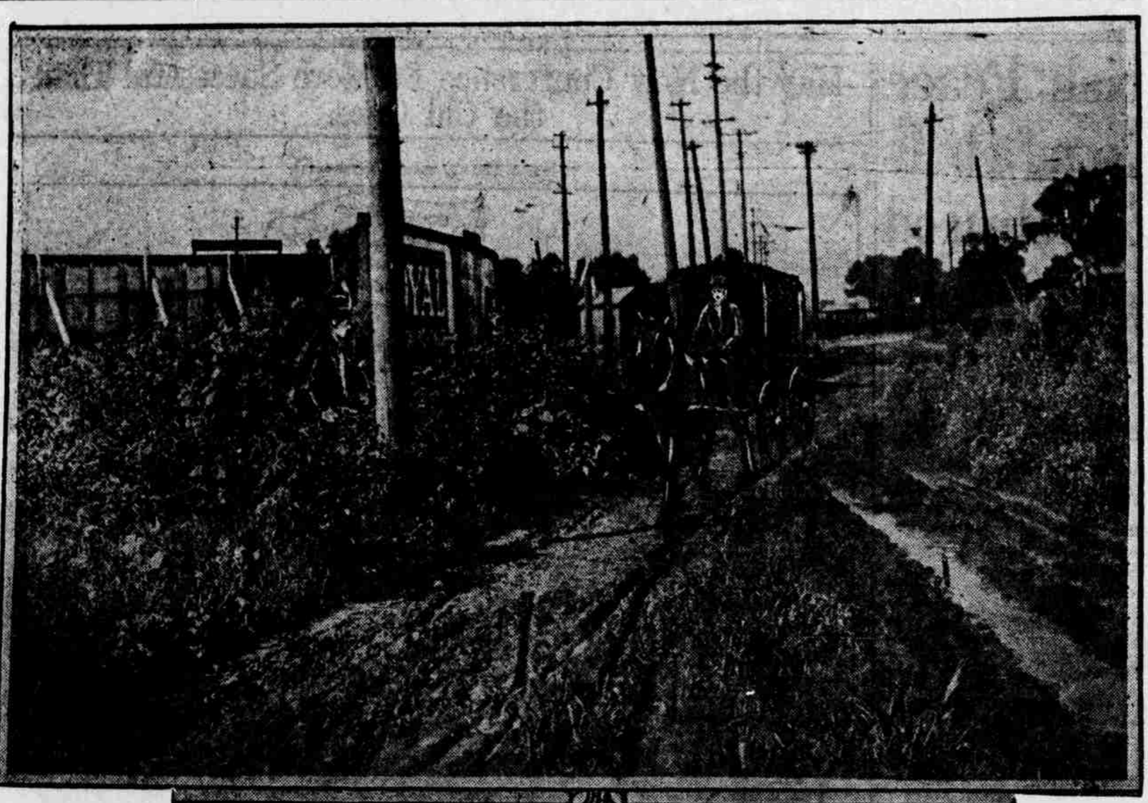
The photograph shows the lonely spot in the road near the intersection of Union avenue with Fifth avenue in Council Bluffs where Walter L. Baldwin, mail driver, was shot down from ambush by an unidentified assassin. The artist has sketched in the position of Baldwin's mail wagon and how the murderer, concealed behind a telegraph pole, fired the shot which brought about his death at 5:25 yesterday morning.
