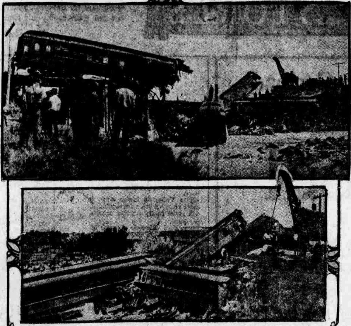
These photographs show how Northwestern train No. 606, bound from Lander, Wyo., to Omaha, crashed through the bridge over Cottonwood creek two miles east of Whitney, Neb., Wednesday night. Five were killed and 32 injured. Baggage car, smoker and chair car plunged into the waters of the creek. The Pullman remained on the rails, as the photographs show.
