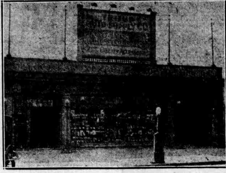
The above picture shows the new location of the Troup Auto Supply company at 2027-29 Farnam street, which affords several times the amount of floor space as the old location at 1921 Farnam street.
