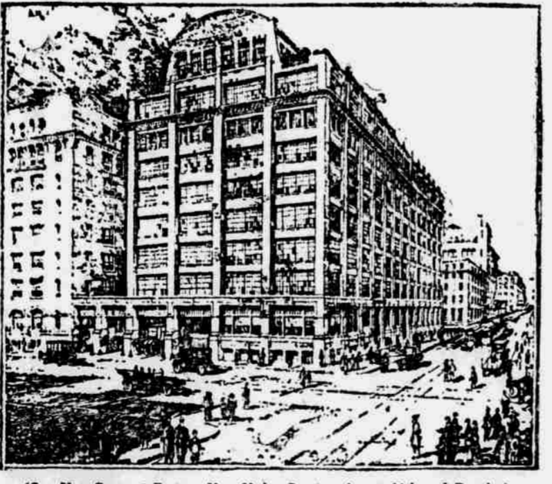
(Our New Garment Factory Now Under Construction at 10th and Douglas)
