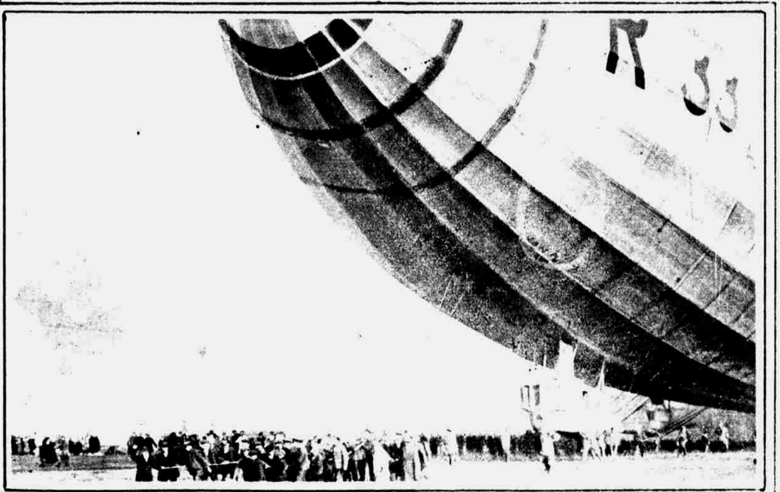
HAULING THE AIRSHIP OUT OF THE HANGAR
