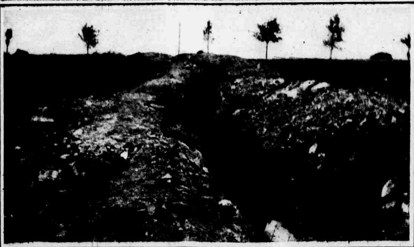
GERMAN FRONT LINE TRENCH SOUTH OF SOISSONS, PHOTOGRAPHED AFTER THE GERMAN RETREAT FROM THE AMERICANS.
