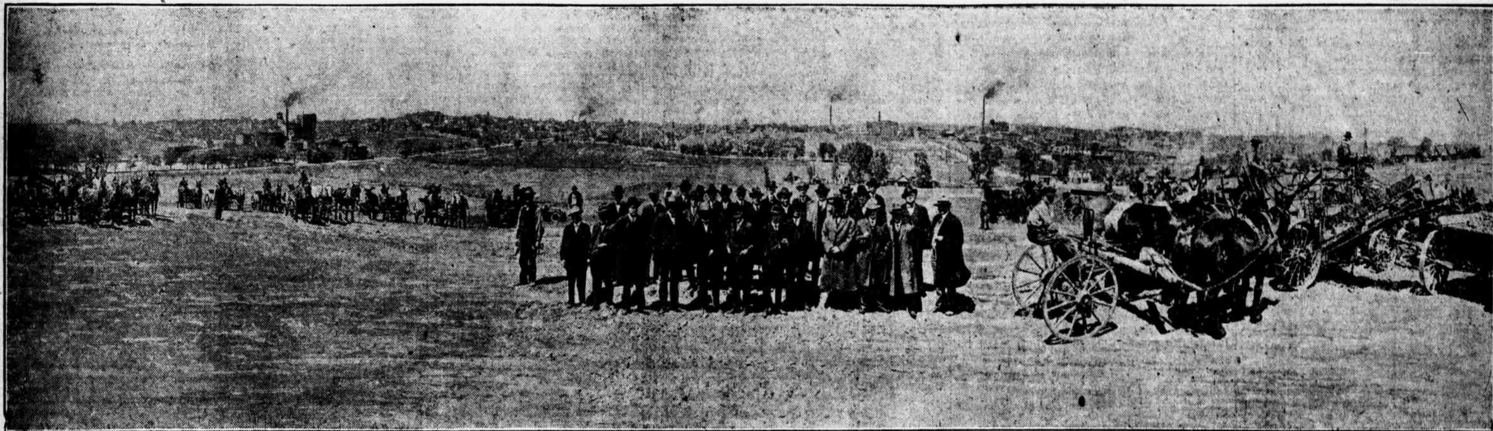
GRADING AND EXCAVATING FOR THE NEW SKINNER INDEPENDENT PACKING PLANT.
