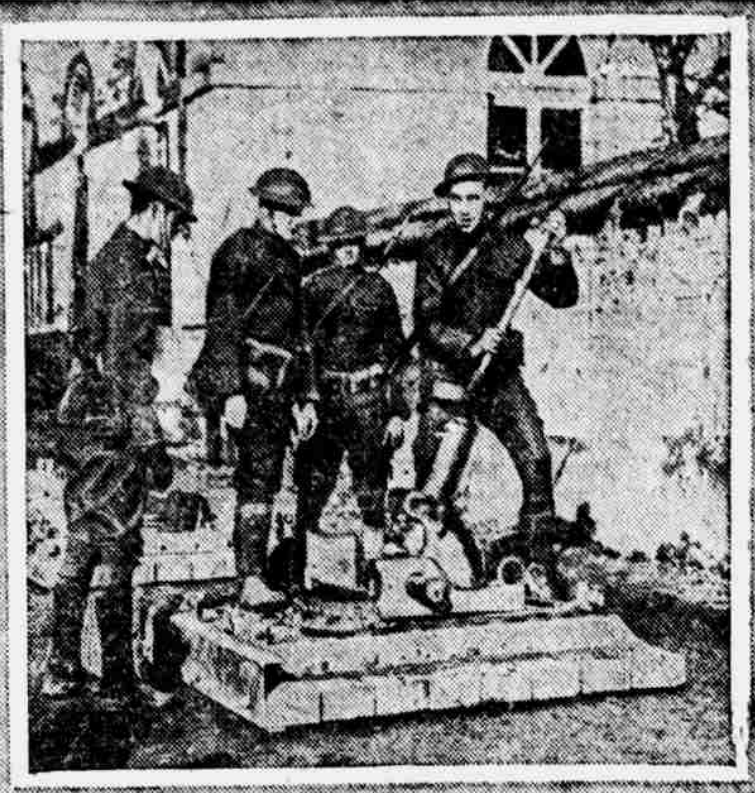
CLEANING TRENCH MORTAR. COURTESY OF THE PACIFIC INFORMATION SUPPLY BUREAU.
