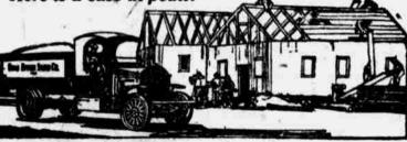
At Camp Taylor, 6 Pierce-Arrows, owned by the Ohio River Sand Company, worked day and night hauling sand and gravel. Every 10 hours they averaged 6 round trips of 12 miles each. No other truck was able to average 5 trips. They carried an aggregate load in less time, with less idle time than any other truck.
