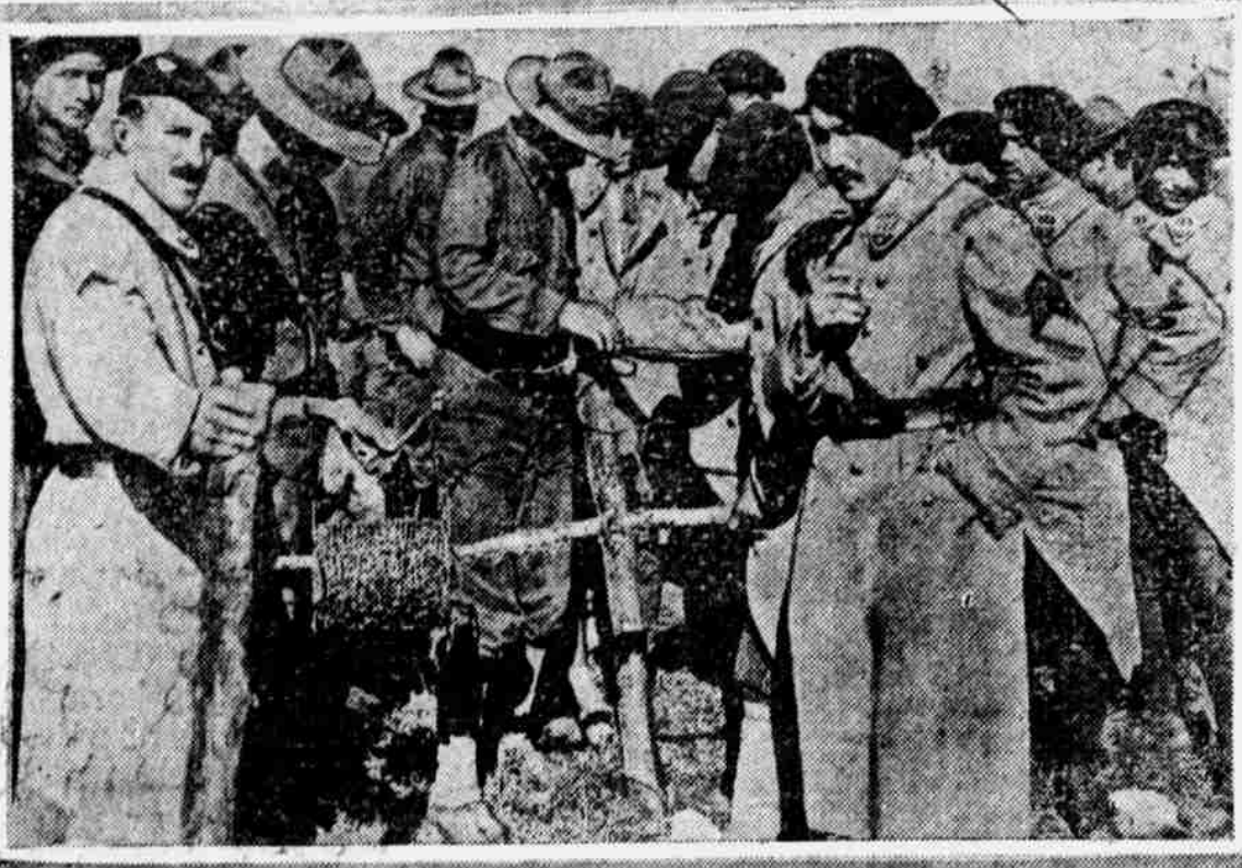
STRINGING UP BARBED WIRE. ©COMMITTEE ON PUBLIC LIBERATION, SUPPLIED BY N.S. French chasseurs instructing our marines in France in the art of erecting barbed wire entanglements.
