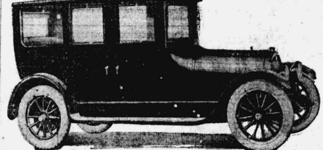
This is one of the classiest jobs that was ever exhibited in Omaha. The body is of the Springfield type, and so constructed so that the glass windows will drop down into the sides of the body and when desired they can be a permanent top and clear vision along the entirely removed and placed in holding the entire length of both sides. These models are brought out eight-cylinder chassis only. This car is now on exhibition sales room of the Apperson to the body and when desired they can be
