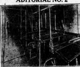
Six Large Combination Pasteurizers and Ripeners Capable of Handling 10,000 lbs. of Butterfat Daily
