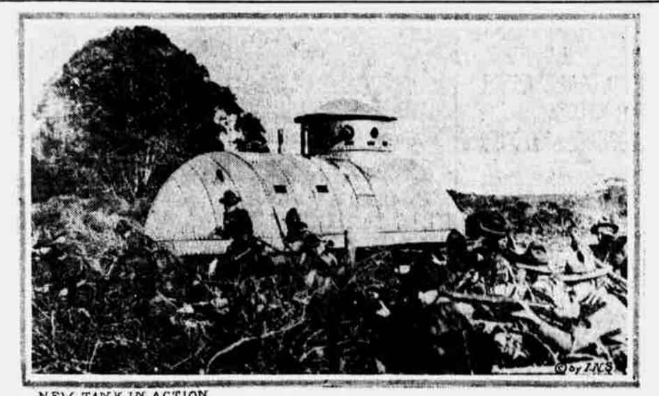
NEW TANK IN ACTION
