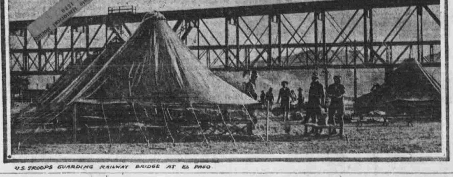
U.S. TROOPS GUARDING RAILWAY BRIDGE AT EL PASO.
