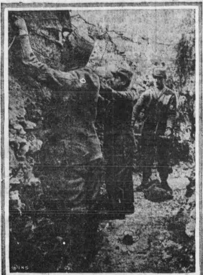
STRINGING TELEGRAPH WIRES IN FRENCH TRENCHES.
