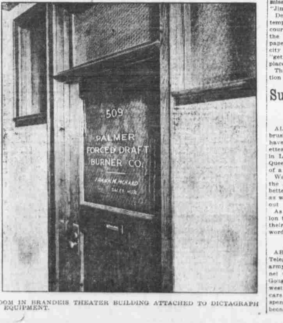
ROOM IN BRANDIS THEATER BUILDING ATTACHED TO DICTOGRAPH EQUIPMENT.
