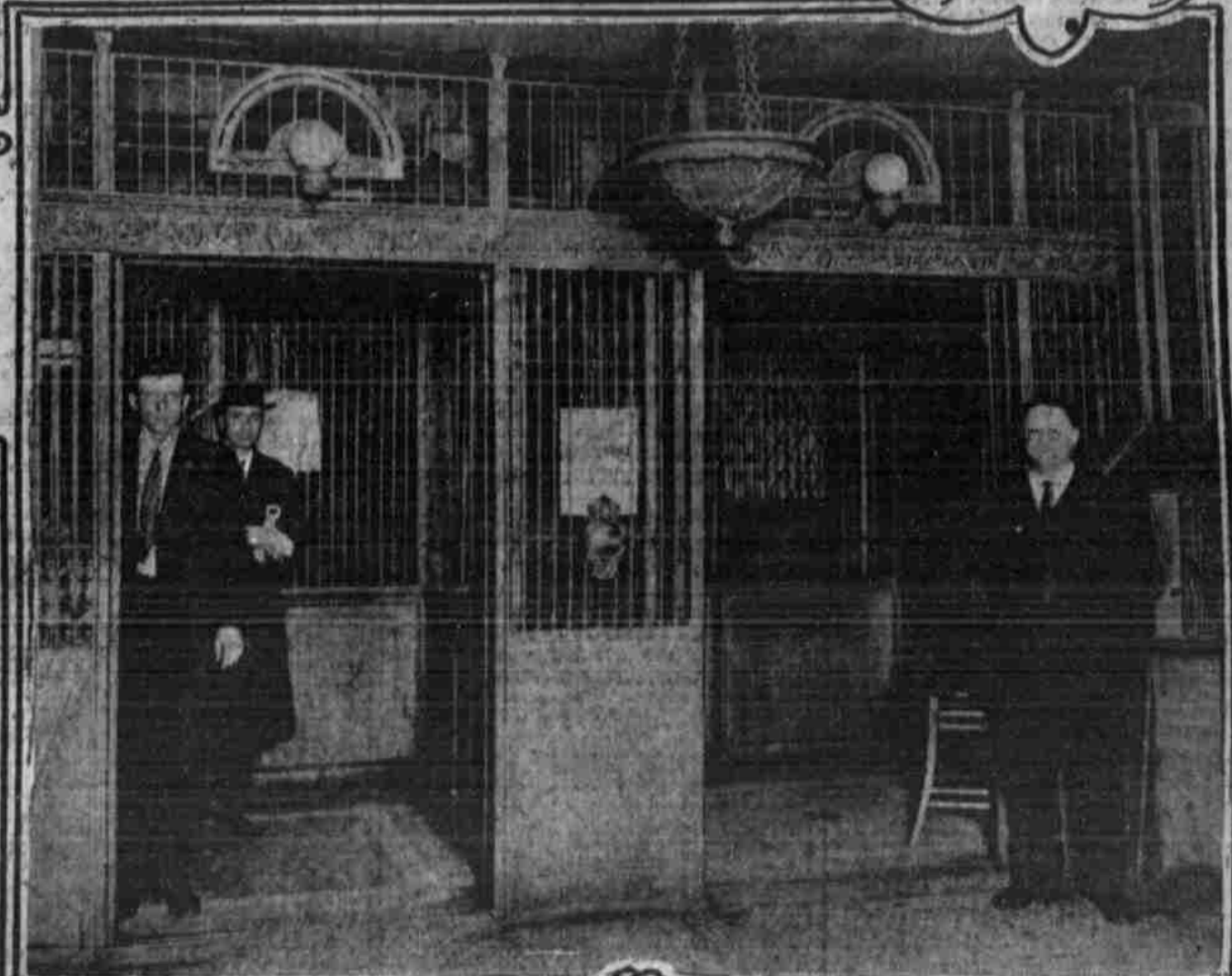
Passenger Elevators in Bee Building
