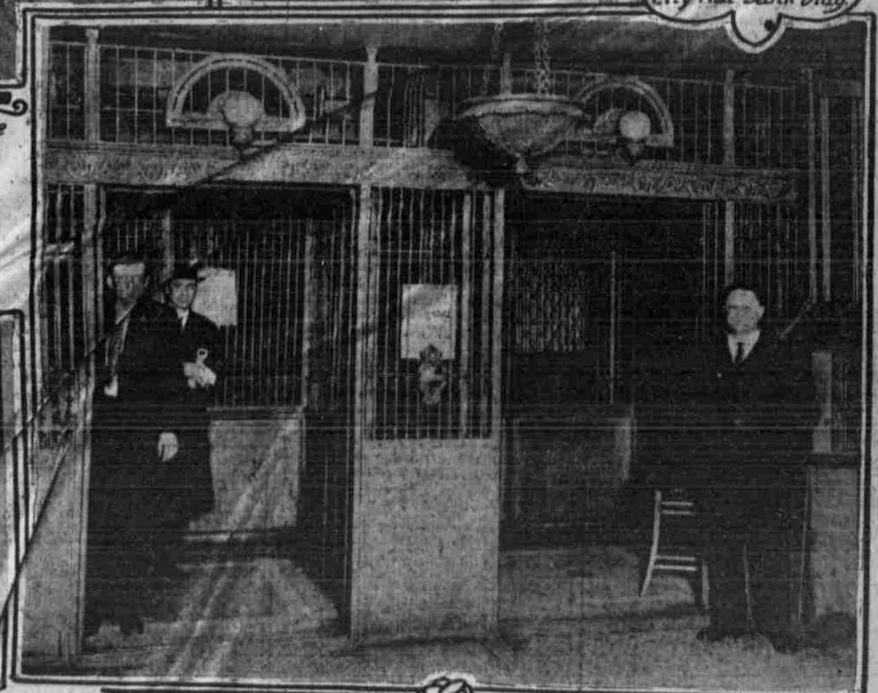
Passenger Elevators in Bee Building
