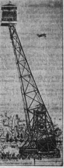
The aeroscope, an inverted pendulun which will have an elevation of 268 feet or four feet higher than the Ferris wheel, Crane arms 240 feet in height, mounted upon a steel tower fifty feet high and made of two parallel riveted trusses, will operate as a balance lever. One of the crane arms carries a double decked cage for passengers at the Panama-Pacific International exposition.
