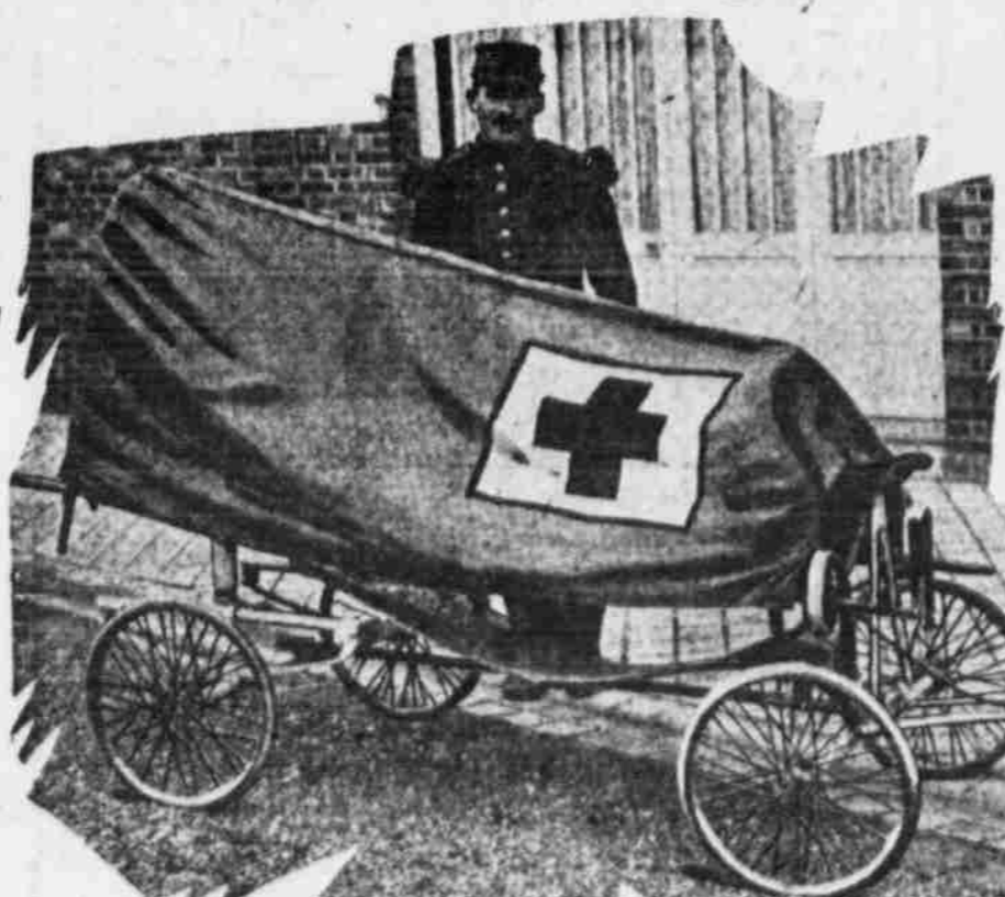
The Small Dog-Drawn Ambulance Designed by Captain Pusais for Carrying a Wounded Soldier from the Field to the Red Cross Hospital.
