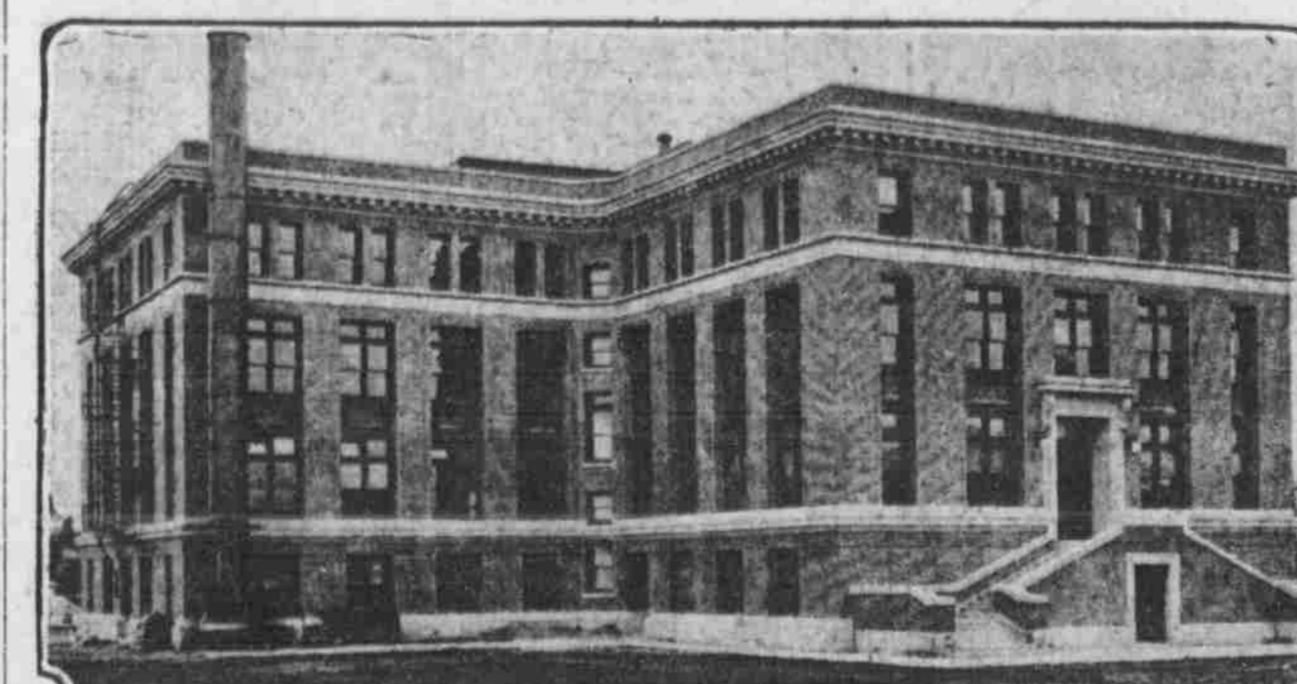
MAGNIFICENT STRUCTURE COMPLETED THIS SUMMER AT FORTY-SECOND AND DEWEY AVENUE TO BE DEDICATED THURSDAY.
