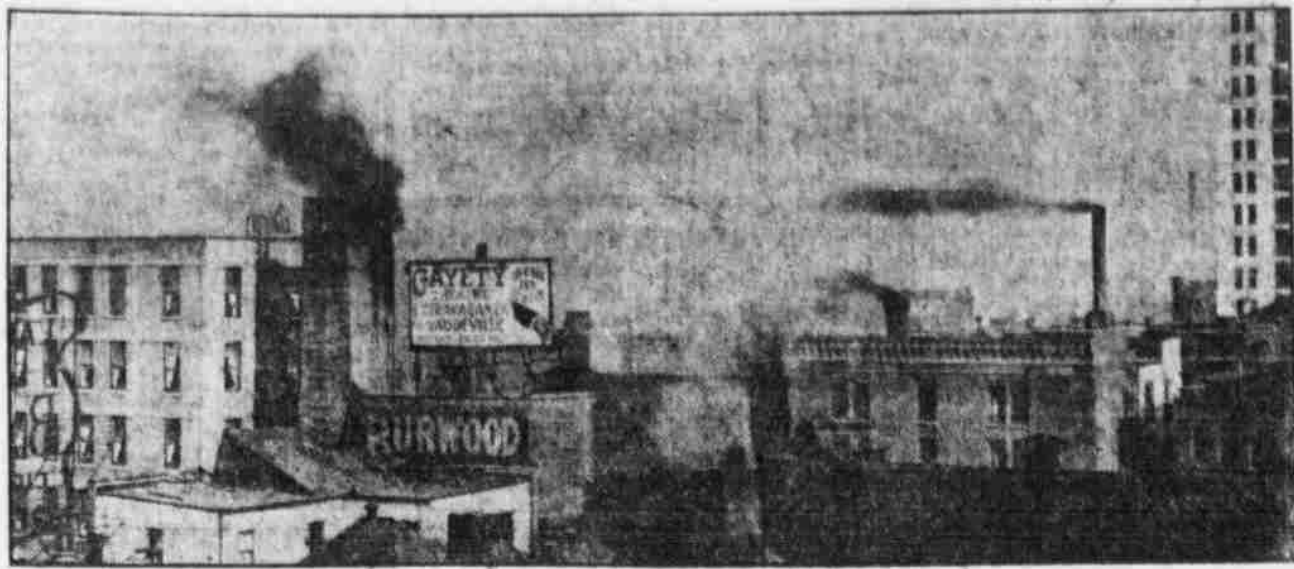
MORE CHIMNEYS POUR FORTH THEIR SOOT AND BLACK SMOKE.
