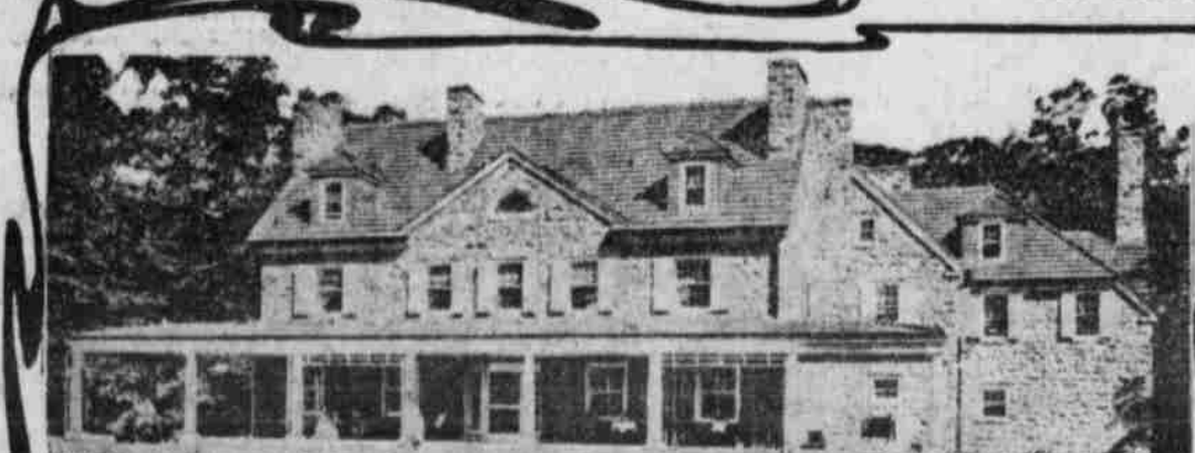
RECENTLY BUILT PENNSYLVANIA HOME
