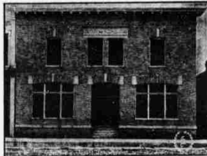
Central City Y. M. C. A. Building
