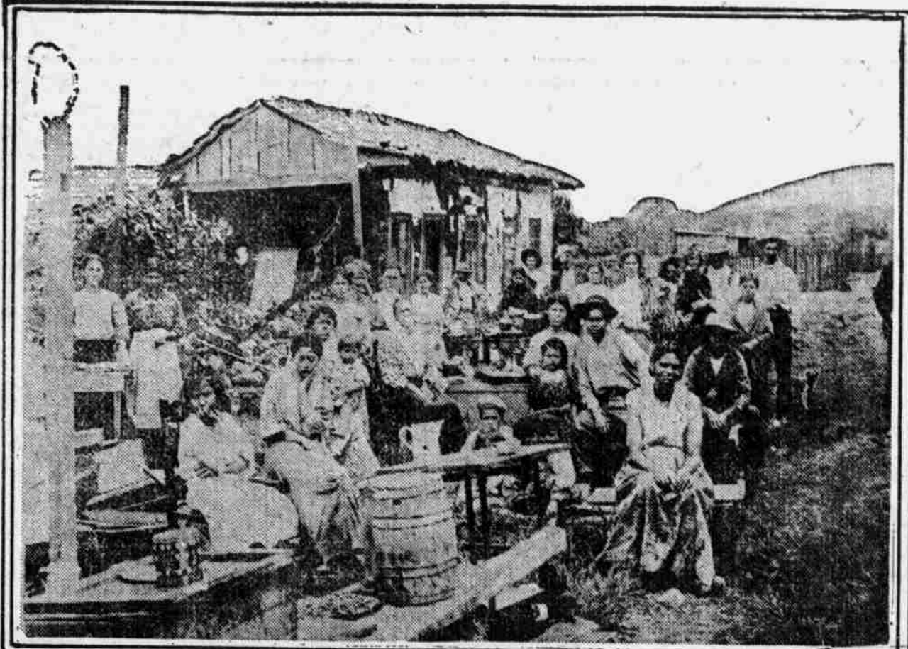
AFTER THE EARTHQUAKE.
