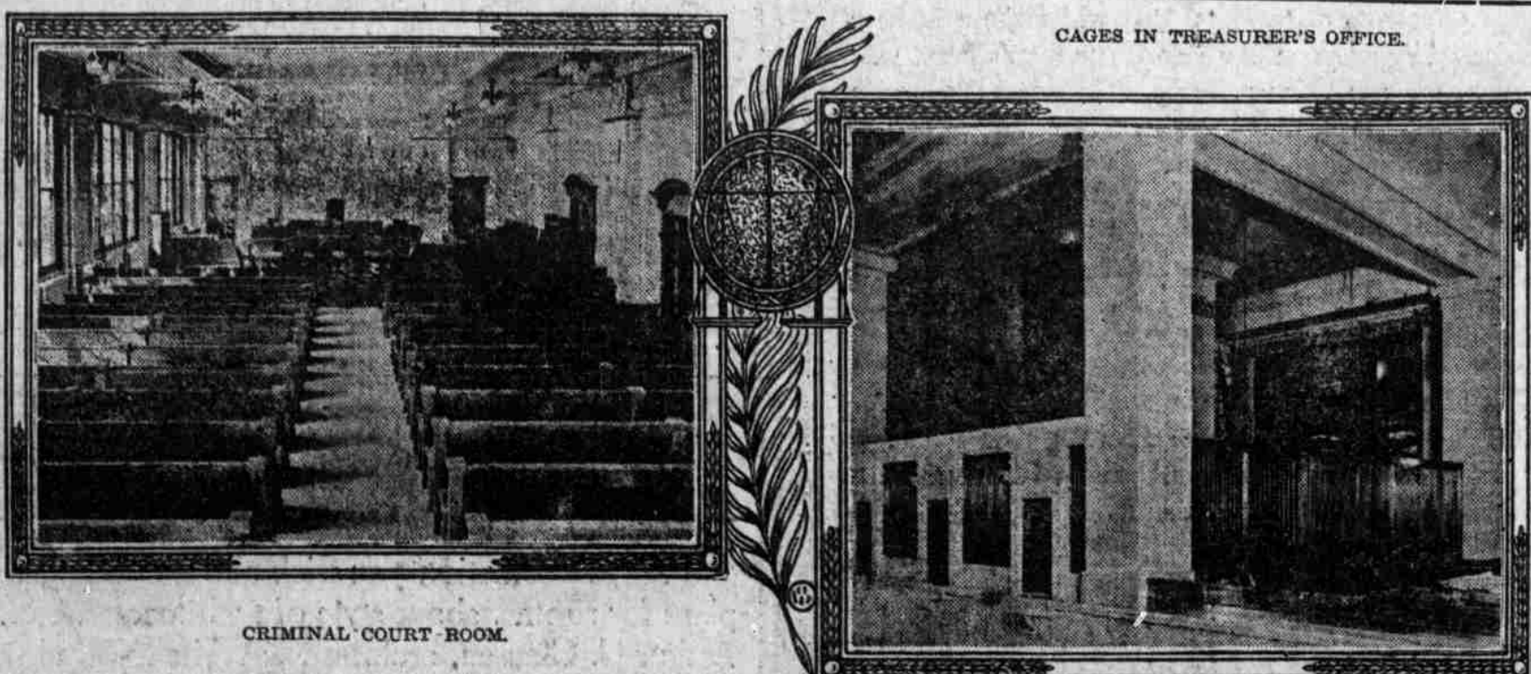
The two interior views presented here of the Douglas county court house, now almost ready for occupation, show the furniture and fixtures supplied by Hayden Bros. The benches, chairs and tables in the court room are of rich quarter-sawn oak. The bars and railings for the cages are of bronze. The furnishings and fixtures are considered to be among the best gracing any public building in the west.
