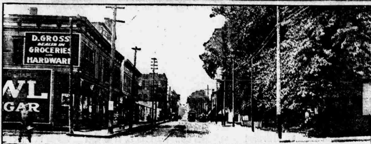
NORTH TWENTY-FOURTH STREET LOOKING SOUTH FROM CHARLES STREET.
