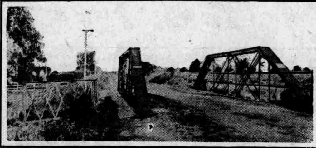
A 60' LOW TRUSS STEEL SPAN ON CONCRETE ABUTMENTS, CONCRETE FLOOR AND SIDE-WALK, IN CENTRAL CITY, NEB.
