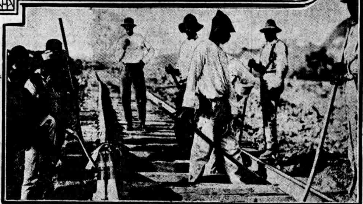
Jamaica Negroes at Work on New Panama Railroad
