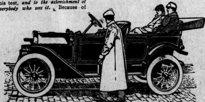
5 passengers—112-inch wheelbase—34 x 4 tires—4 cylinders, 4 x 4 1/2—dual ignition system, with magneto-top—gas tanks and lamps—all included (f. o. b. Dayton).
