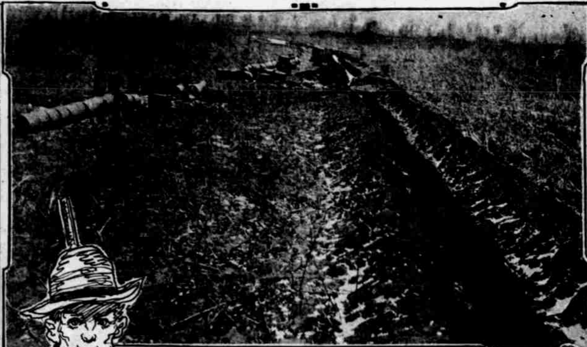
Ditches and Tile Work
