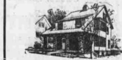
A No. 1-12-W IDEAL Boiler and 415 ft. of AMERICAN Radiators, costing the owner $175, were used to heat this cottage. At this price the goods can be bought of any reputable, competent fitter. This did not include costs of labor, pipe, valves, freight, etc., which are extra and vary according to climatic and other conditions.
