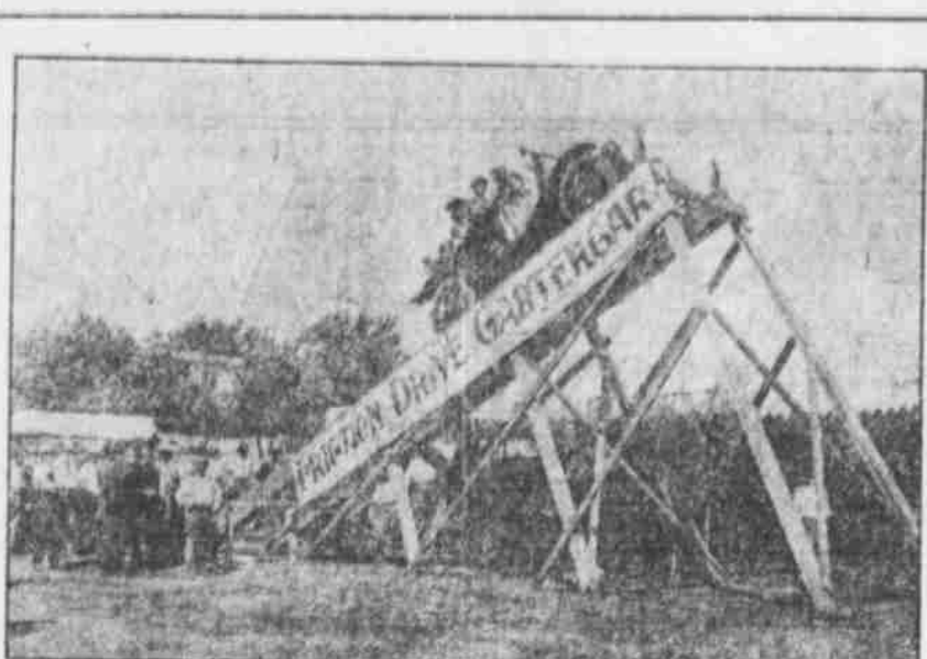
EXHIBITION DAILY AT THE LAND SHOW. The Carter climbing automobile in the Machinery hall at the Land show each day is doing what it is claimed no other automobile can do—that is, climb an incline of 45 degrees. The Carter car climbs the incline with as much ease as an ordinary car would go up an incline of 10 degrees, backing down onto the level without any apparent effort. There is no hour of the day that a crowd is not around the Carter show exhibit, watching the performances of the machine.
