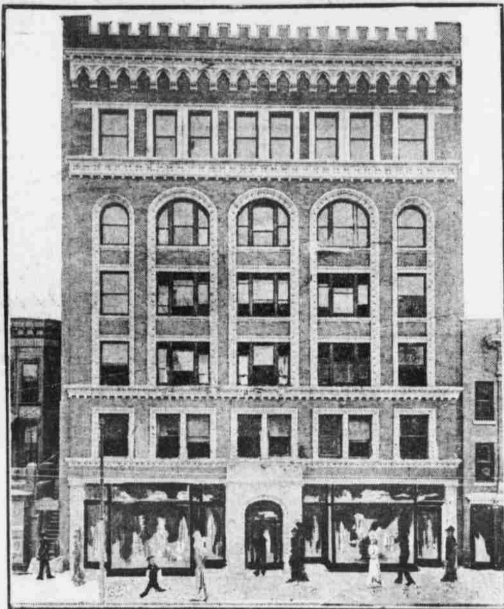
The new Wellington, built at a cost of over $1,000,000, is modern in every particular. The entire interior construction of steel girders carried on iron columns, there being no supporting partitions whatever. The building is semi-fireproof in its construction, all floors being laid in concrete and asbestos plaster board, wire lath and metal studding being used. All floors and halls are of tile, the entrance and first stairway of white marble. A circulating system of hot water supplies every room in the hotel. The building is equipped with the automatic sprinkler system. The entire rear of the building on the alley will be provided with a magnificent stair fire escape.
