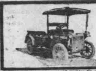
OMAHA ELECTRIC LIGHT & POWER CO. OMAHA, NEB.
