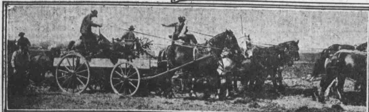
Loading Gumbo from Elevating Grader
