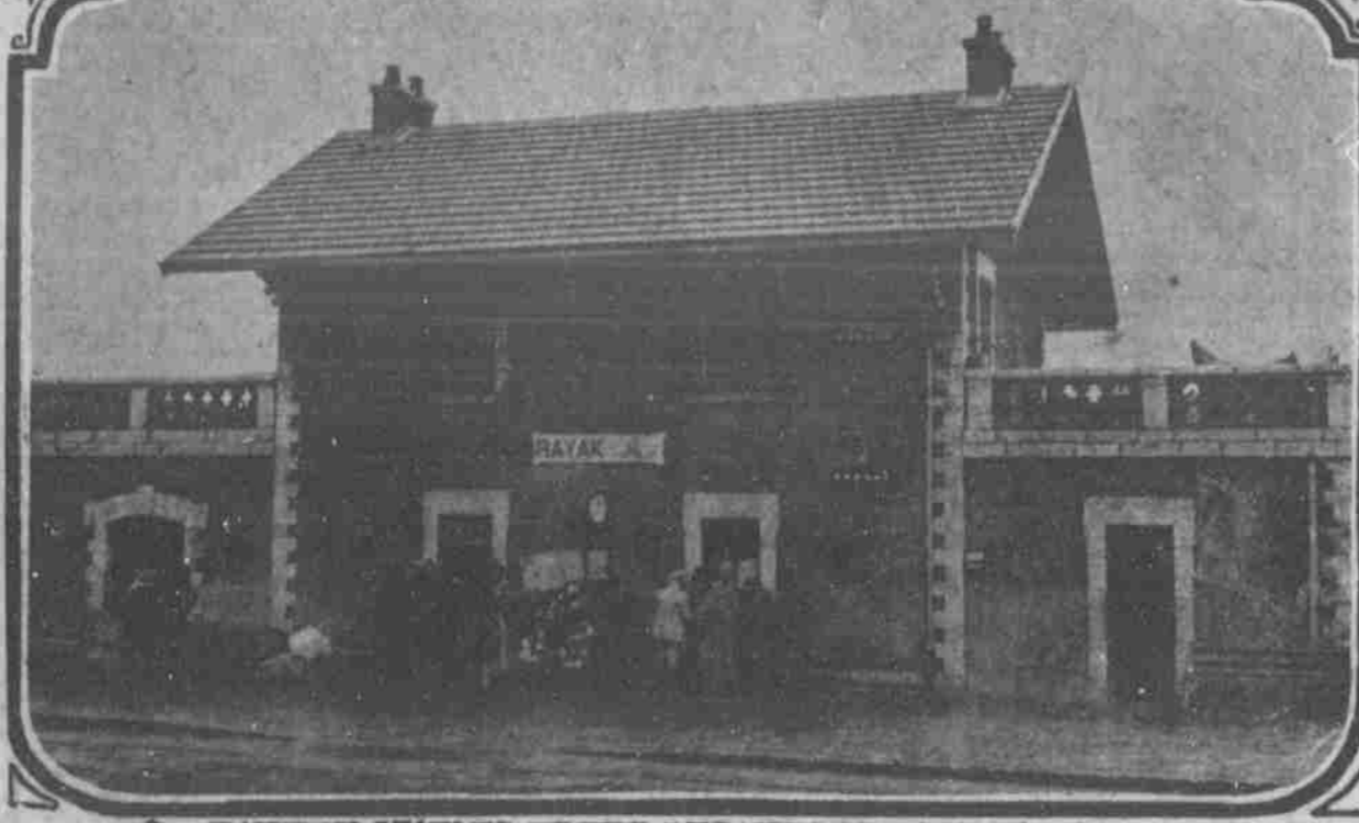
RAILWAY STATION IN THE LEBANON MOUNTAINS
