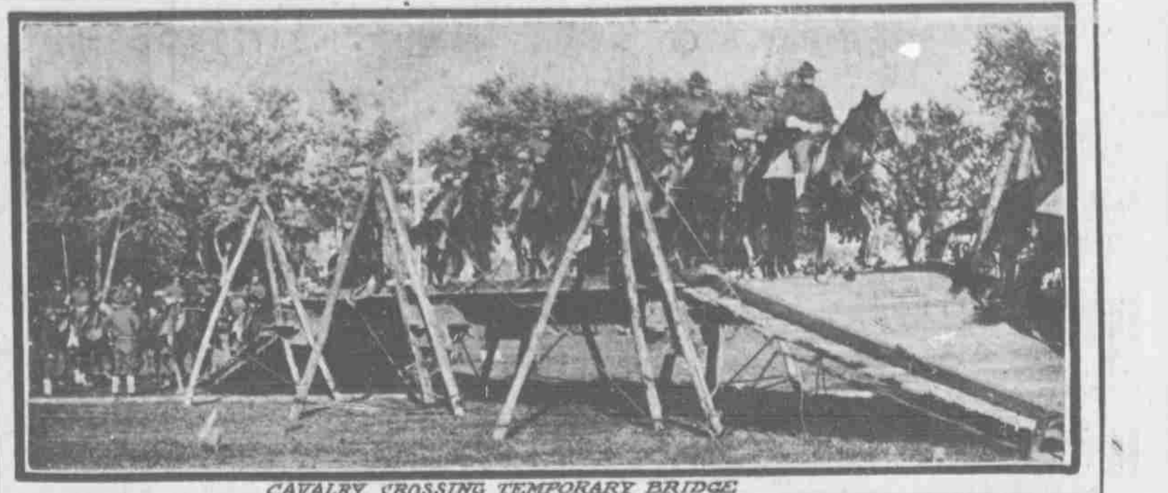
CAVALRY CROSSING TEMPORARY BRIDGE
