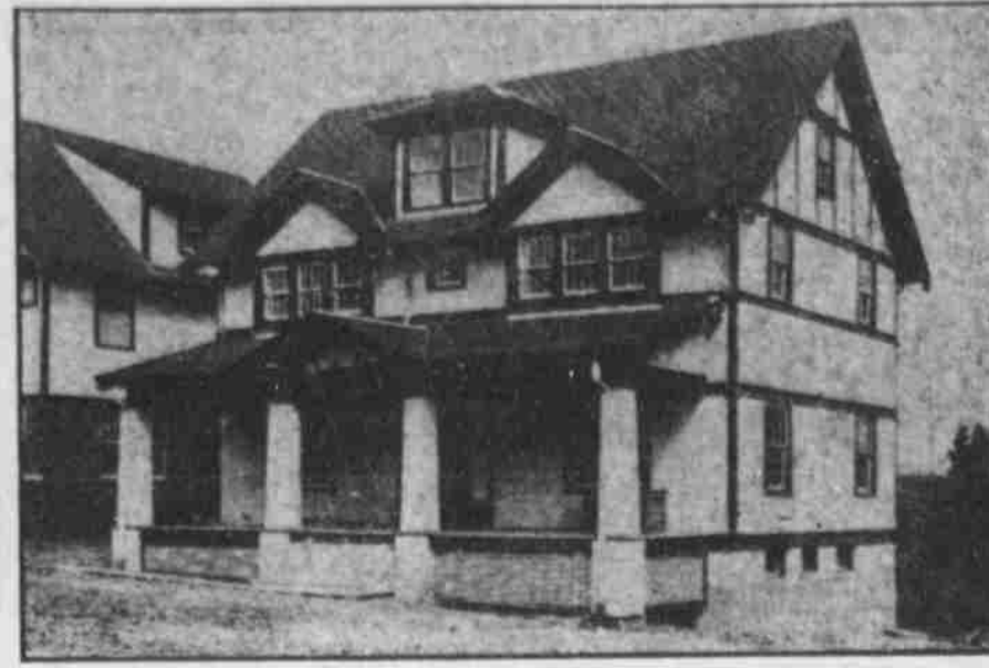
THIRTY-EIGHTH AVENUE DAVENPORT STREET.
