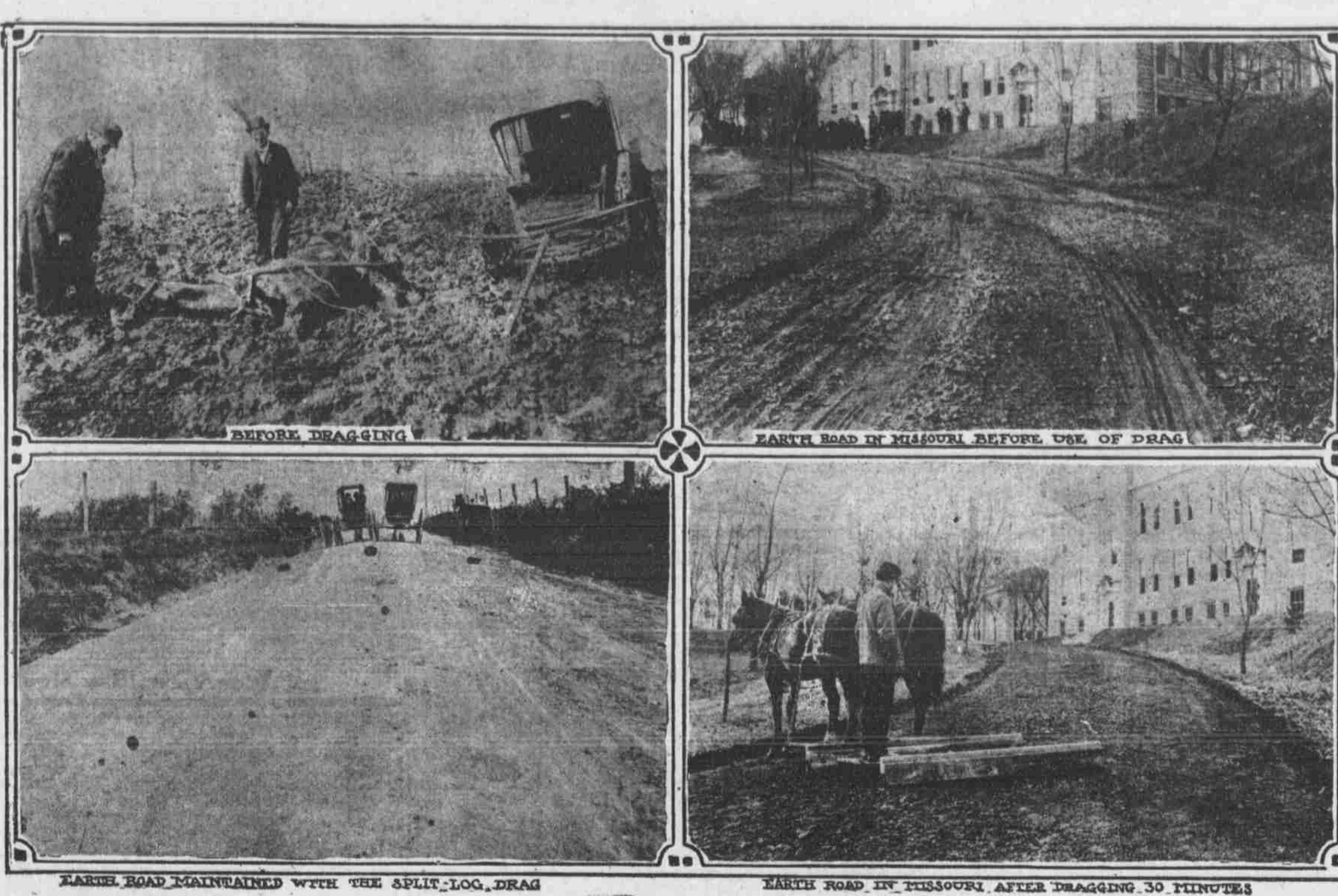
EARLY ROAD MAINTAINED WITH THE SPLIT-LOG DRAG
