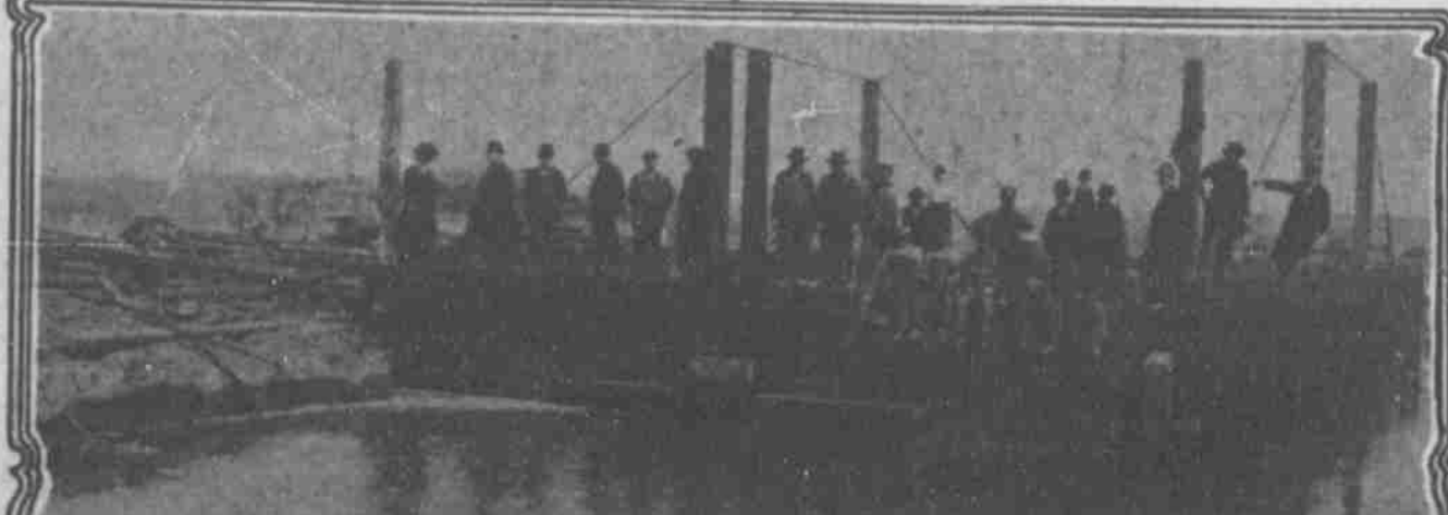
BIG DREDGE BARGE FOR THE PAPHILLION DRAINAGE CANAL
