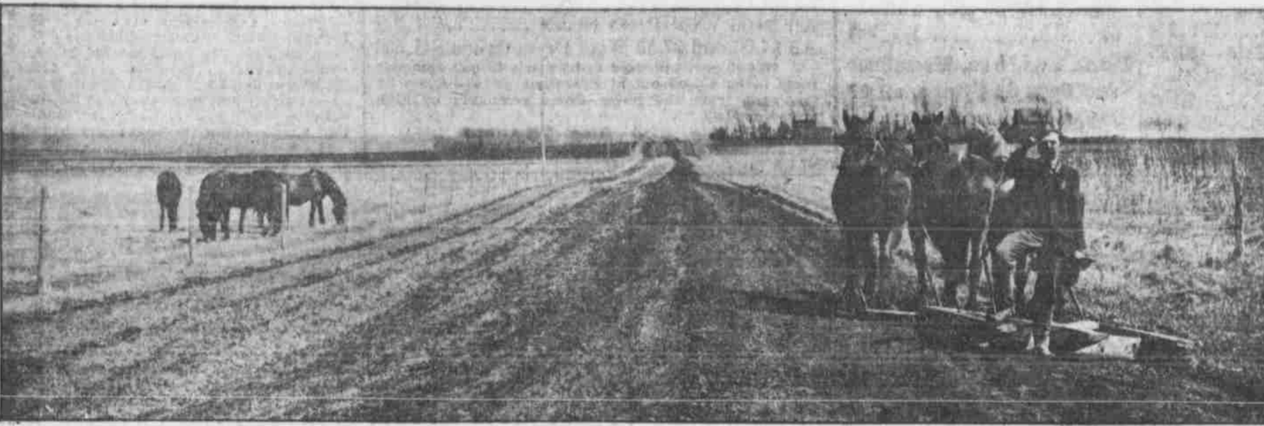
WELL CROWNED ROAD THAT SHEDS WATER AND IS SMOOTH AS A FLOOR.
